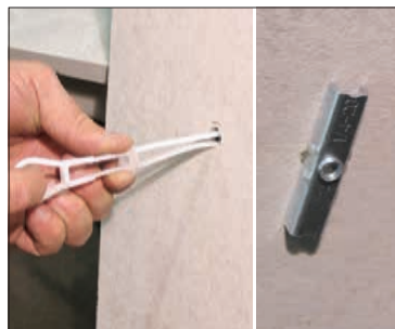
STEP 2 Pull back and slide keeper along ratchet
